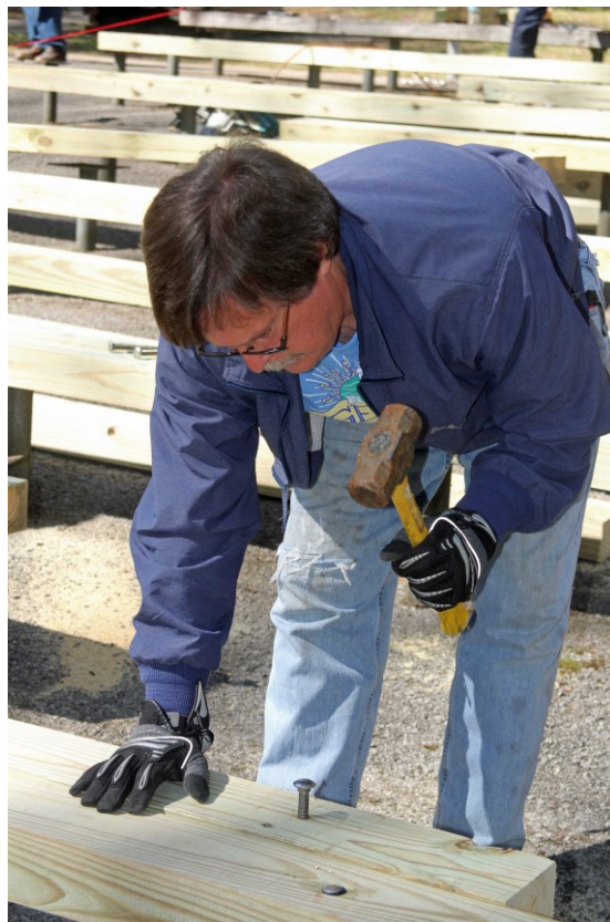
George Dailey hammers the bolt home to secure the bench seat
